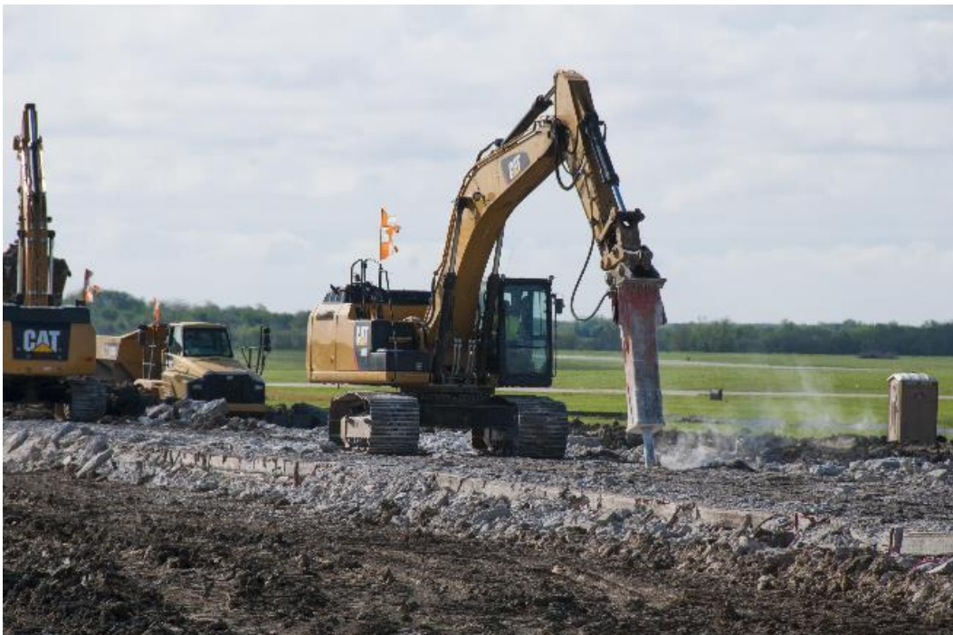
Figure 22: Typical concrete pavement demolition operation using percussive hammer breakers
