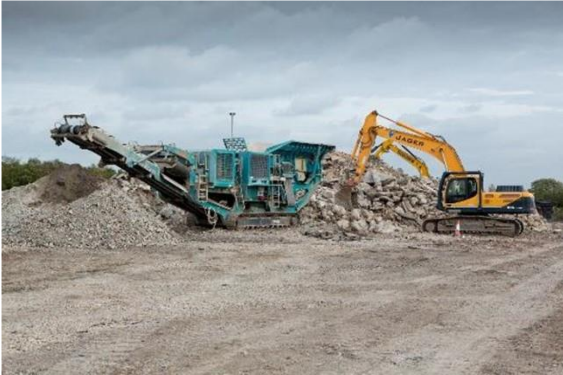
Figure 33: Example of site-based crusher arrangement (Old Oak Common Crossrail Depot)
