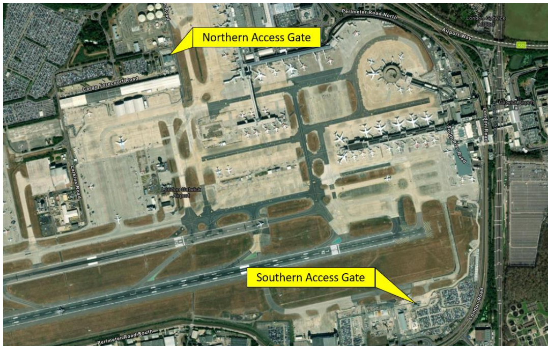
Figure 3737: Locations of North and South Access Gates
